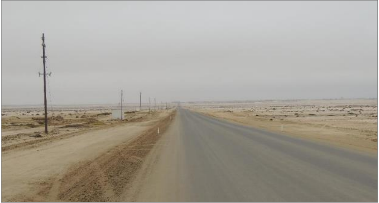
Figure 9: View southwards towards Swakopmund on the C34 National Road
