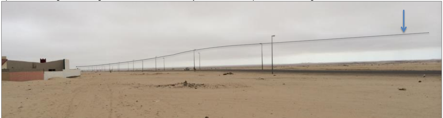
View of probable above ground routing as seen from Swakopmund northern residential
