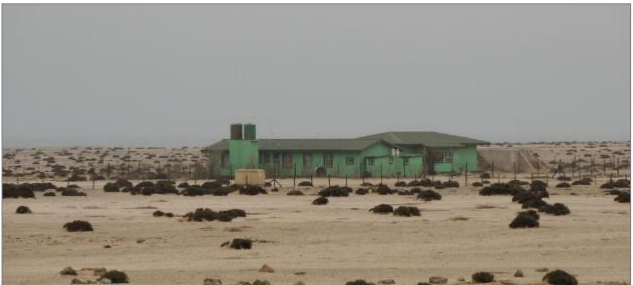
Figure 11: Photograph of the Guano Company structures (top) and the green house as seen from the C34 road
